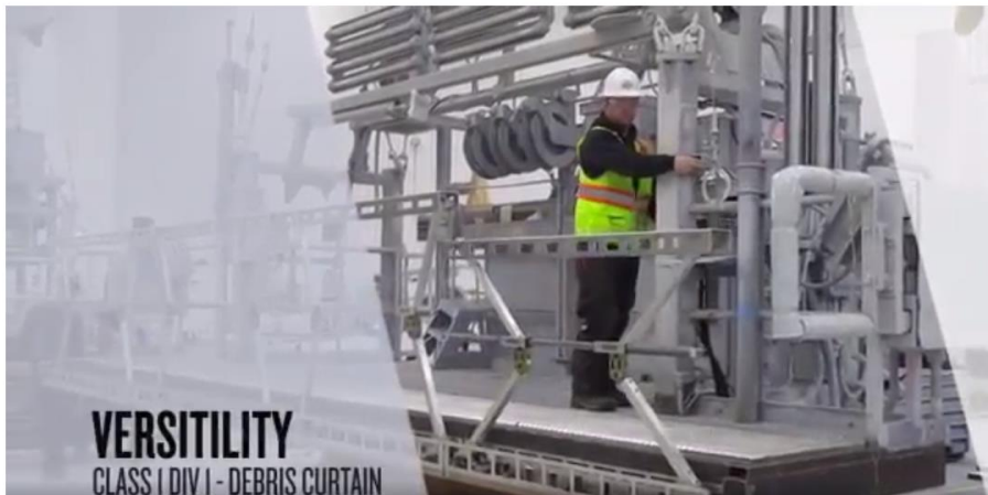
Pneumatic System in Hazardous Paint Environment
